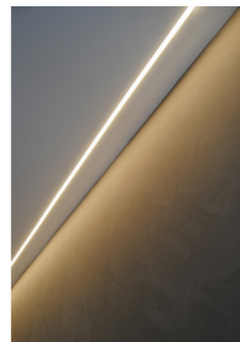
LED Strip Lighting
